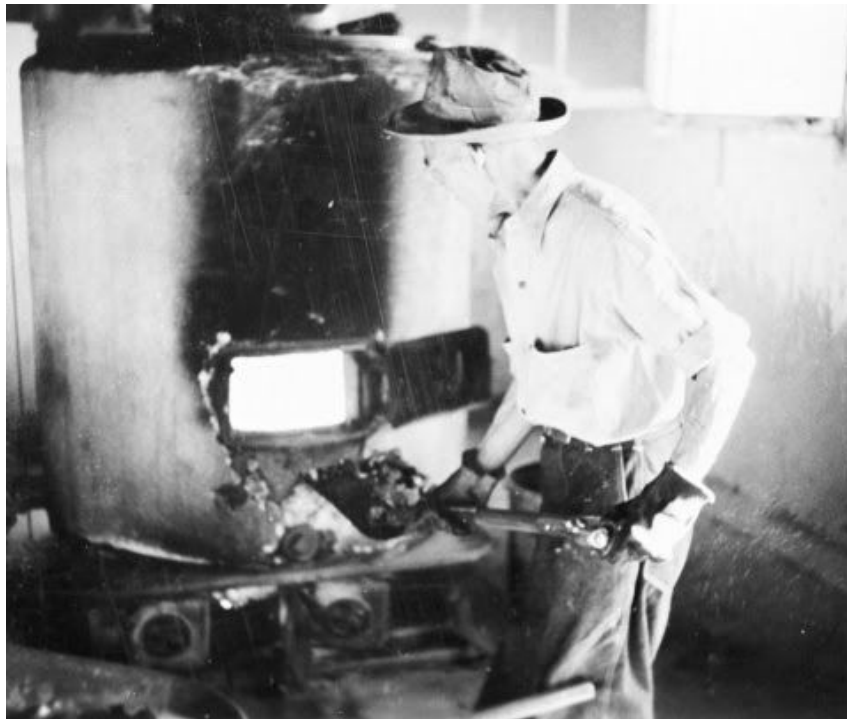
Camp inmate shoveling coal into the block's central heater, which will warm water for the laundry and bath facilities. Photo taken at Minidoka c. 1944. Courtesy of the Mitsuoka Family Collection, Densho.
