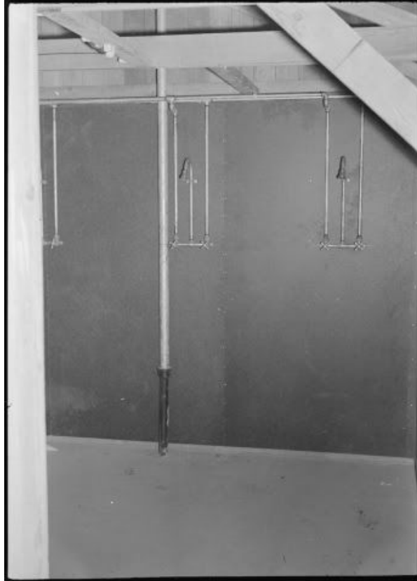
Shower facilities at Poston. May 3, 1942. Photo by Fred Clark, courtesy of the National Archives and Records Administration.
